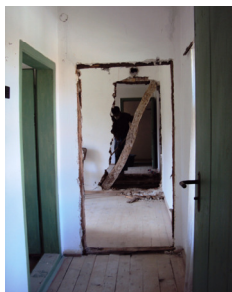
The upstairs hallway now reaches all rooms.
