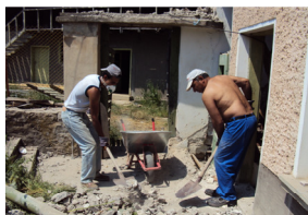
Kamil and Akif removing the outside stone staircase.
